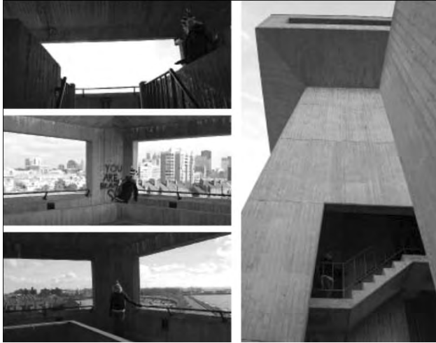
Figure 9. Photographic series of “A look out the observation tower” depicting the concrete enclosed staircase and the open panoramic views.
